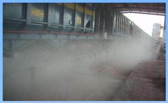
**Pre-Wetting DS System – Waiting Wagons** The Fogging type spray nozzle fitted on the entrance of the receiving pit area will spray to moisten the top layer at the wagon.
